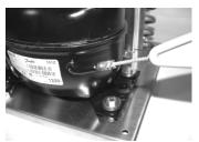
covering the compressor discharge tube (closest to the label) and use the round wire tube/fitting brush (079-2001) to clean the inside of the compressor discharge tube. Only twist the round wire brush clockwise. Use the abrasive cleaning pad to clean the shoulder of the discharge tube on the compressor.
