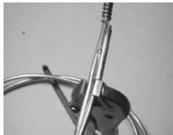
8. Before flaring the ends of the evaporator lines for attachment to the base valves, insulate the lines with the tubing insulation (055-0036) to prevent sweating. Cap the ends of the tubing before sliding the insulation over the tubing to prevent any foreign matter from entering as the tubing slides through the insulation.
