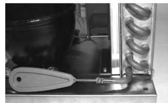
28. Solder this connection using preparation procedures mentioned previously in the Preparation Section. After the tubing has cooled, adjust it so the filter-drier (020-0500) is centered in the saddle mount (400-0900) and the bends are a good fit around the base. Thread the flare nut (027-0001) onto the discharge base valve (096-0040) and tighten firmly with two wrenches.
